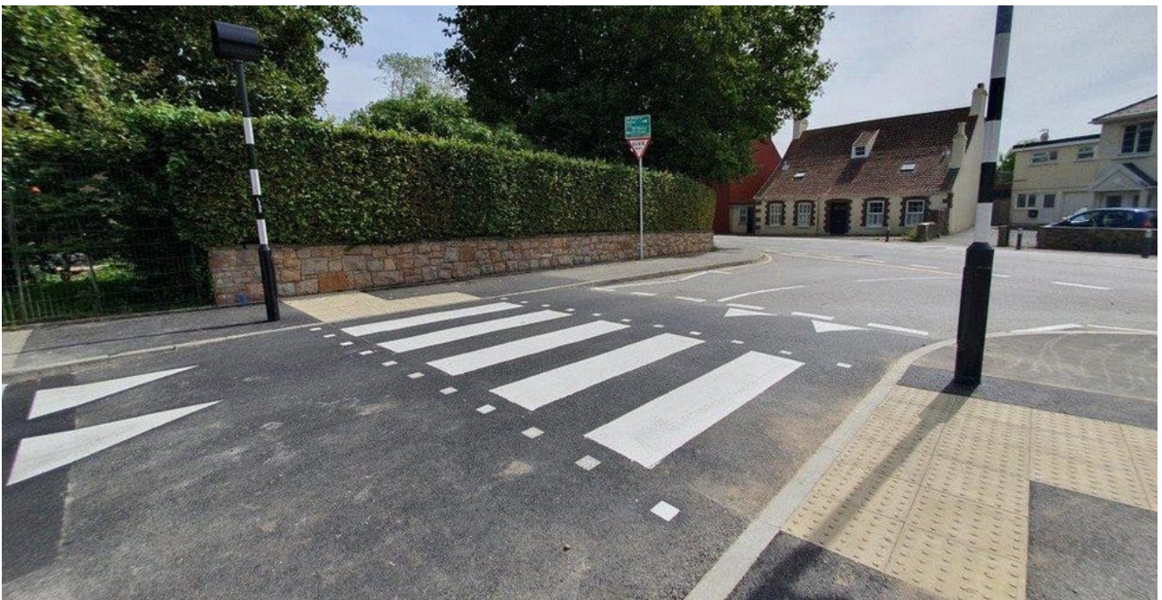
Figure 6-2: Raised table crossing points
