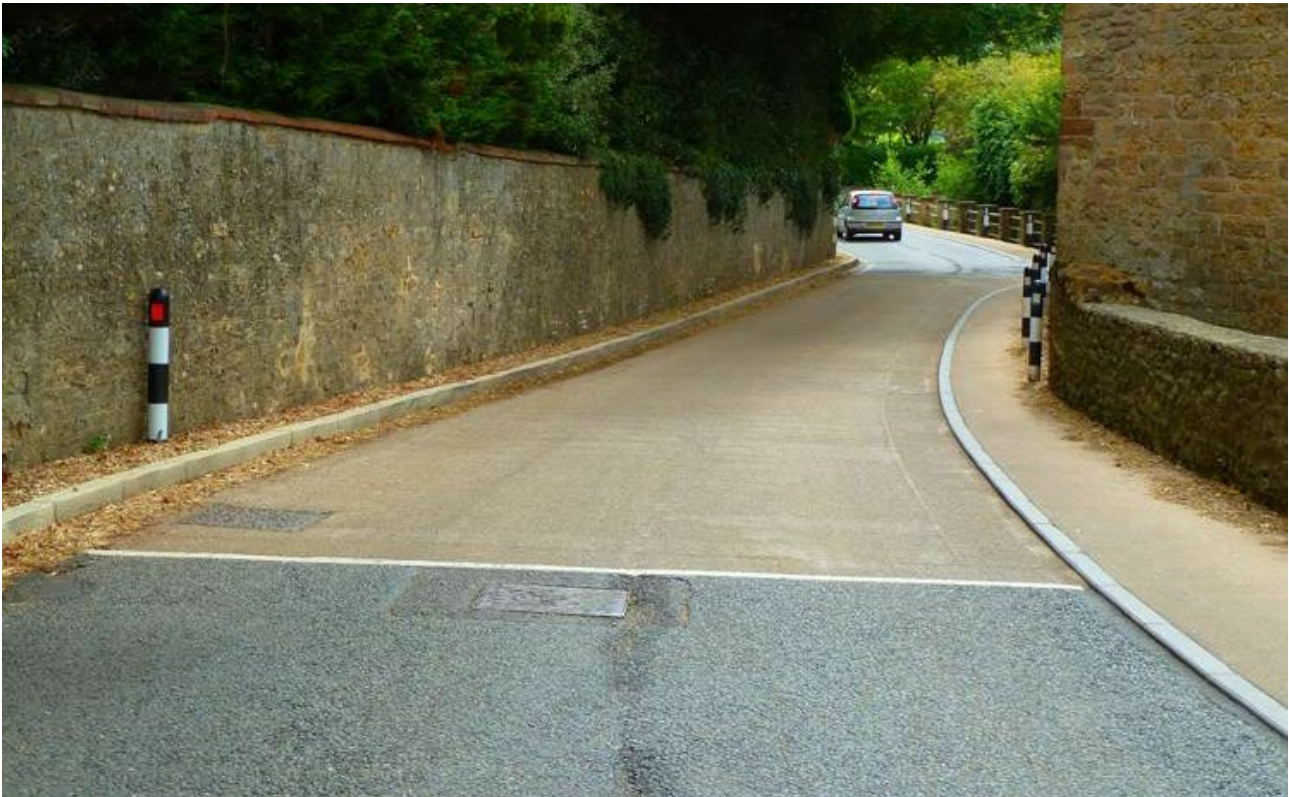
Figure 6-4: Removal of white lines/surface treatment
